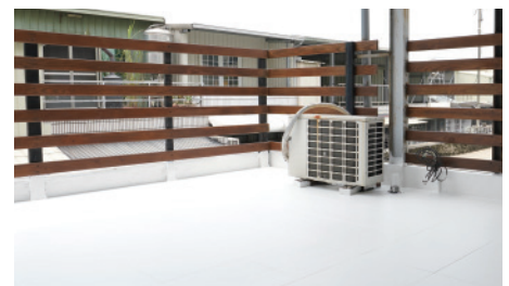
Photo of Lock Roof Water Based Waterproof Coating Application
