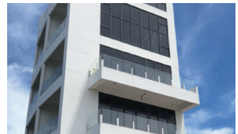
Photo of Water-based Dirt Resistance Elastic Paint Application
