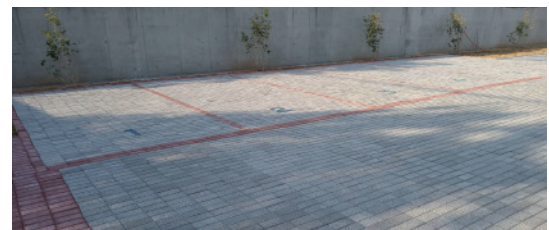
High-Pressure Permeable Concrete Block applied to outdoor parking lot.
